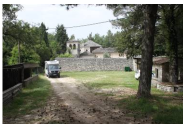
The entrance to the site with the monastery in the background
