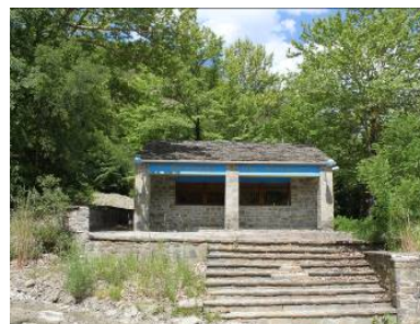
Building across the site with fresh water and toilets
